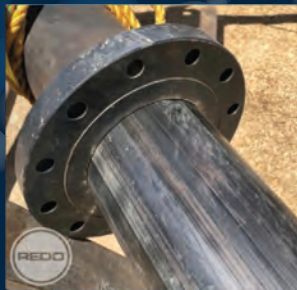
Tight Fit Lining
