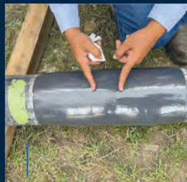
Non-Metallic composite overwrap repair (NCO)
